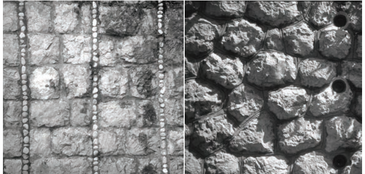
Vila "Vesna" Detalj kamene obloge, SI zid, Lopud, Hrvatska, Nikola Dobrović, 1939 Vila "Vesna" Detalj kamene obloge, JZ zid, Lopud, Hrvatska, Nikola Dobrović, 1939 Ljubaznošću Krunoslava Ivanišina Villa Vesna, Stone cladding, detail, NE wall, Lopud Croatia, Nikola Dobrović, 1939 Villa Vesna, Stone cladding, detail, SW wall, Lopud Croatia, Nikola Dobrović, 1939 Courtesy: Krunoslav Ivanišin
